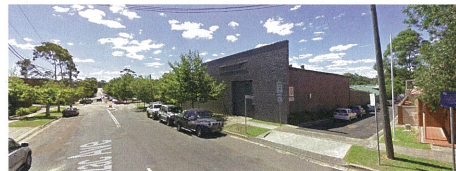
View from South East Corner
