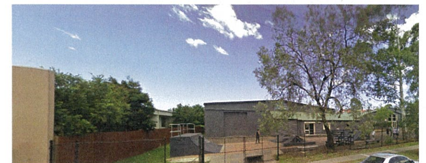
View from North West Corner
